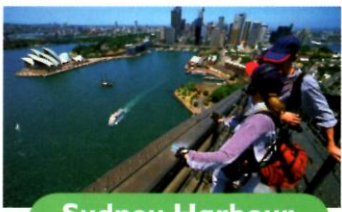
Sydney Harbour Bridge
